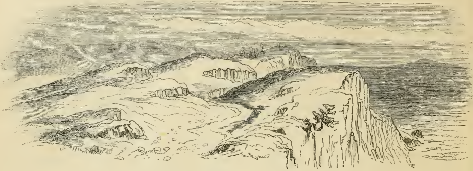
Course of the Wall at Caerboran, looking over the Moss.
